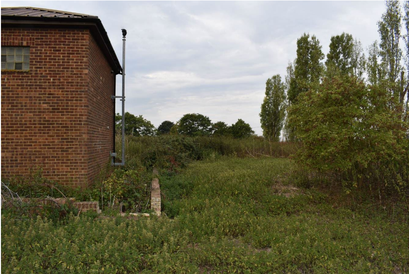
Plate 13: Rear of the existing borehole building (facing W)
