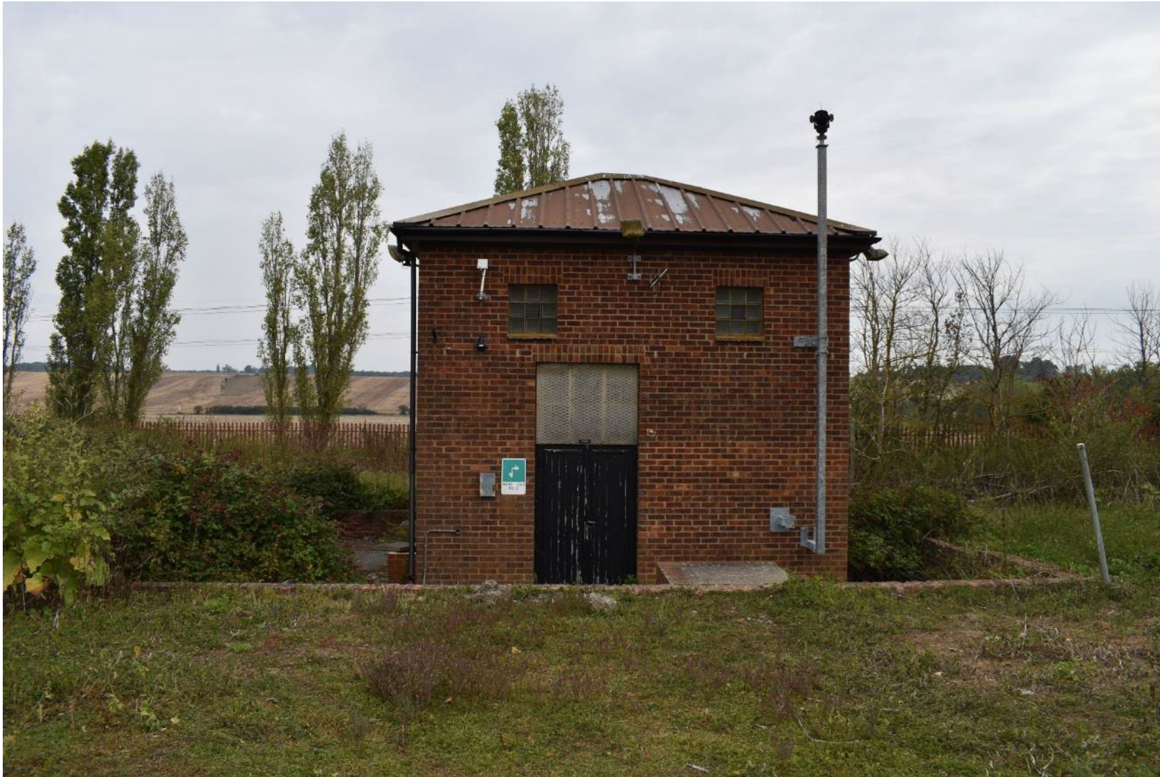
Plate 12: View of the existing borehole building (facing N)
