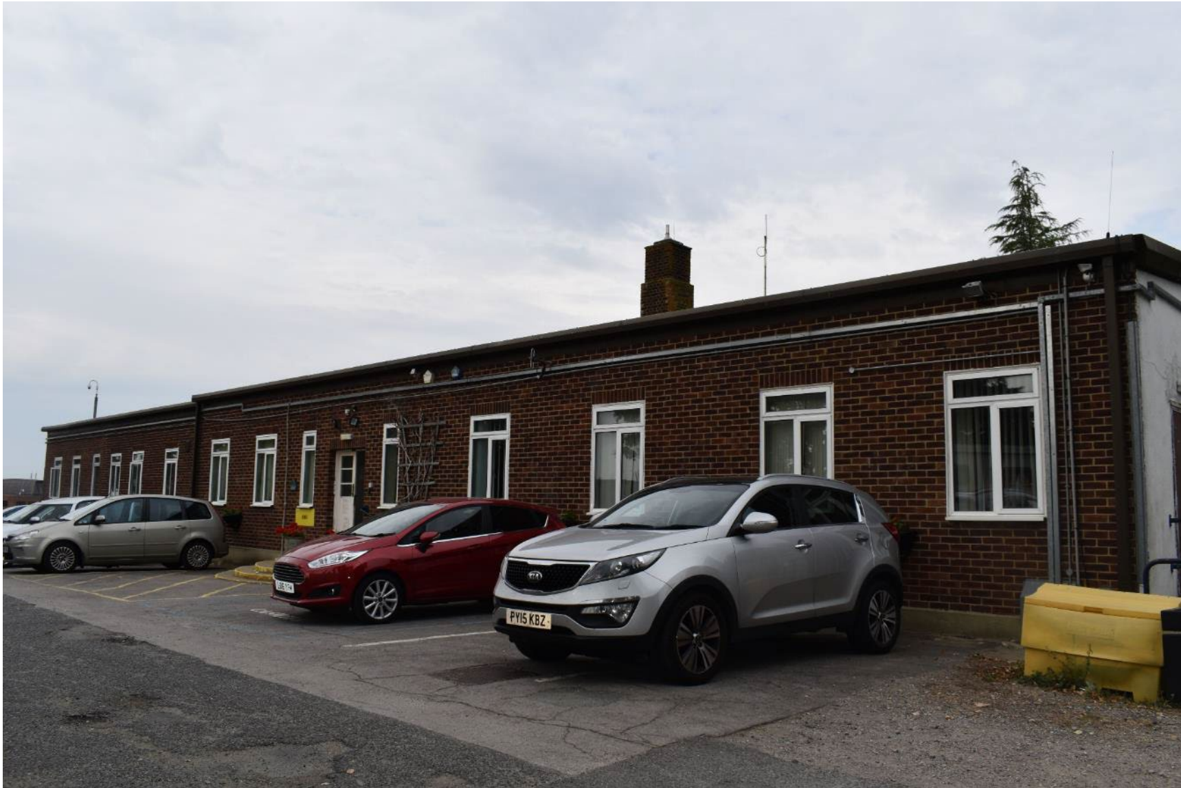
Plate 22: Existing admin building (facing SW)
