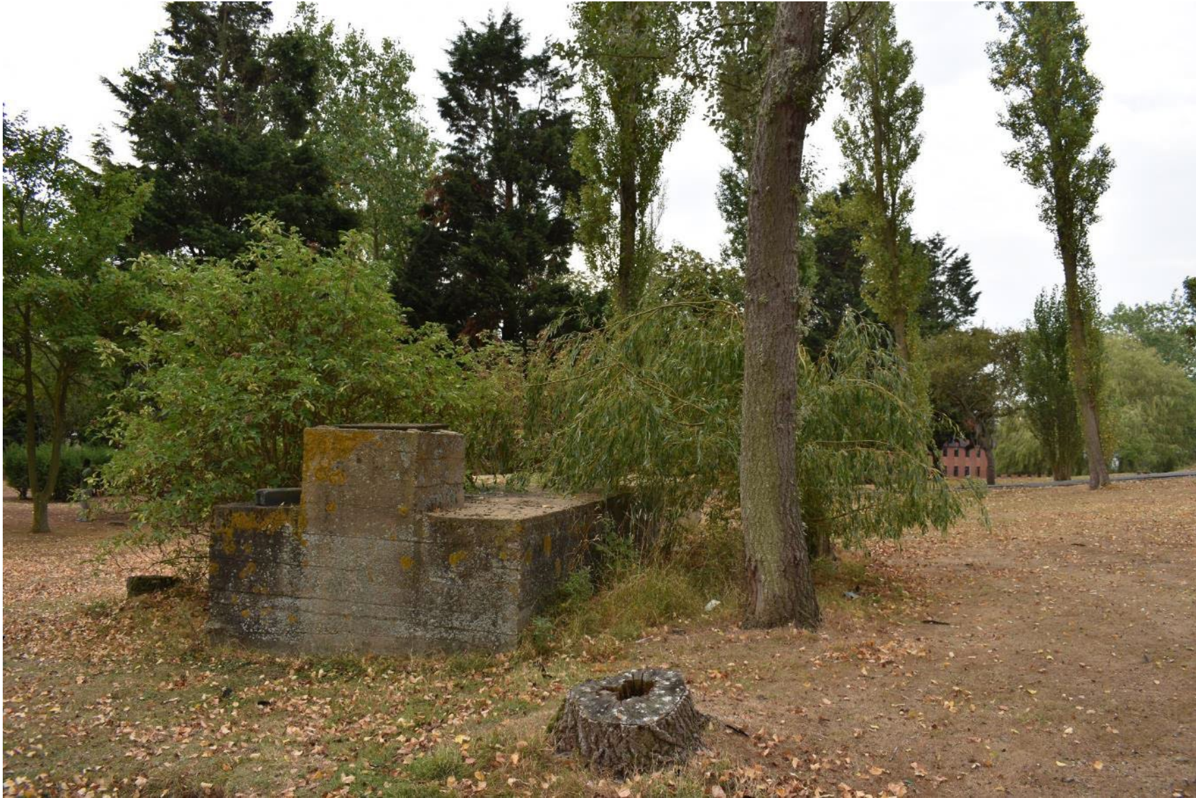
Plate 19: Rear view of the World War II bunker (facing SE)
